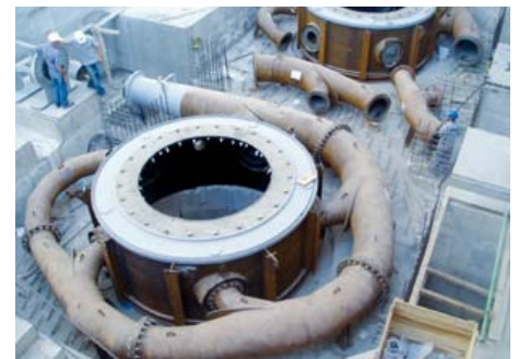
LAMAS IV HPP, Turkey 2 vertical 5 nozzle Pelton D_1 = 1,210 mm P = 2 \times 10.8 MW, H = 325 m
