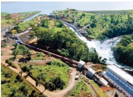
IRARA HPP, Brazil 3 horizontal Francis D_2 = 1,650 mm P = 3 \times 10.5 MW, H = 31.5 m
