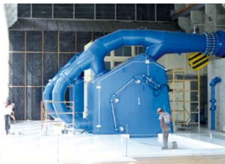
LAS VACAS II HPP, Guatemala 2 horizontal 3 nozzle Pelton D_1 = 1,310 mm P = 2 \times 10.7 MW, H = 285.6 m
